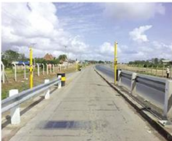
Mariakani HS-WIM; Left: A truck shown a Green Light is compliant and continues on its journey. Right: Truck is shown a Red Light is not compliant, it is diverted to the Static Weighbridge. Currently all the weighbridges in Kenya are being managed by SGS
