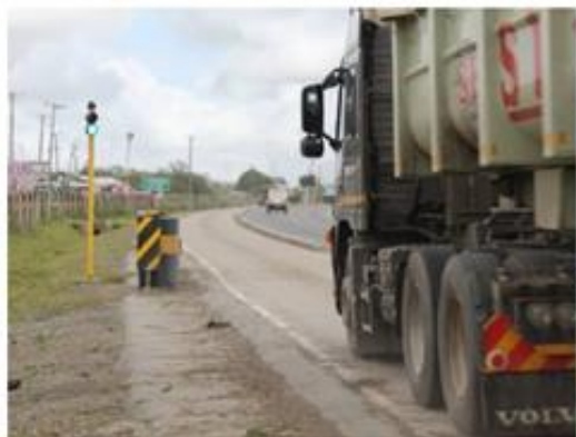
Mariakani HS-WIM; Left: A truck shown a Green Light is compliant and continues on its journey. Right: Truck is shown a Red Light is not compliant, it is diverted to the Static Weighbridge. Currently all the weighbridges in Kenya are being managed by SGS
