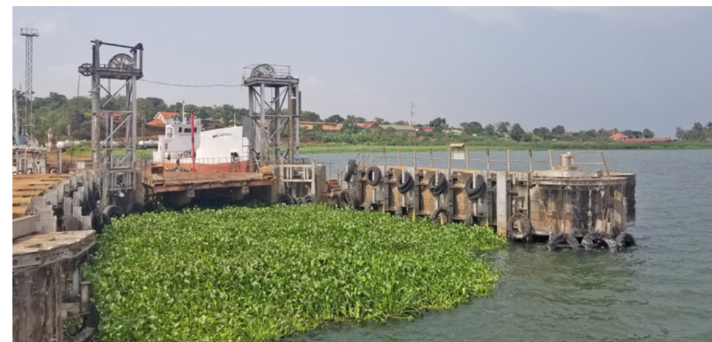
Figure 18: Linkspan guide walls with worn-out fendering
